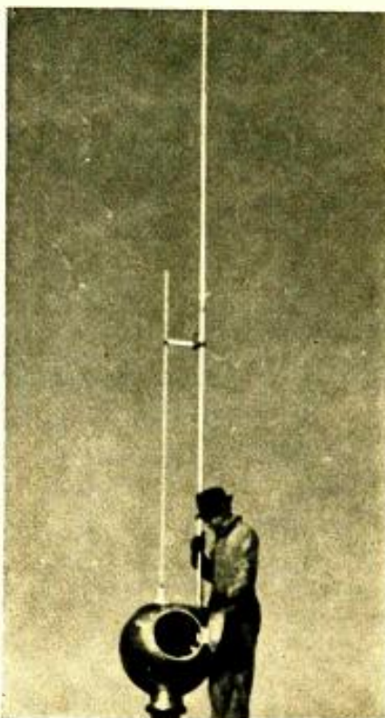
The W8XNT "J" type antenna, 758 feet above ground, atop the Terminal Tower building in Cleveland.
